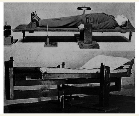
Figure 9 Mosso's balance (top) and its modified version (bottom) built by Lowe at King's College London (adapted and reprinted with permission from Lowe, 1936).
